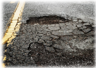
INDIAN ROAD PROFILE BROKEN SURFACES
