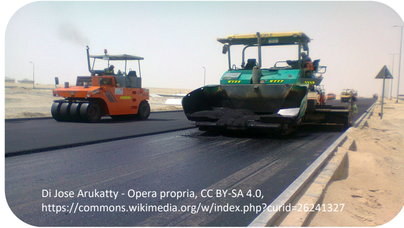
Re-surface test tracks
